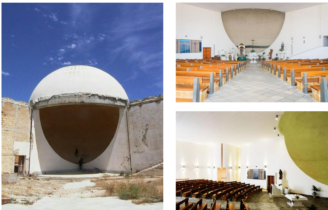
Figure 2. The interiors, before and after the collapse
