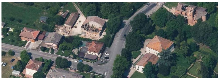
Figure 2. Medolla, Modena. The roof, resting on long span walls, collapsed and directly contributed with its thrust to the out-of-plane overturning of the walls.
