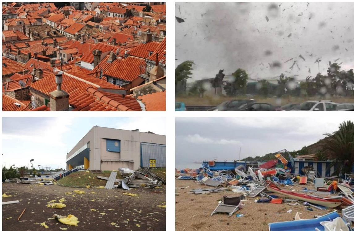
Figure 3. The context assessment is essential to identify the possible risks and the elements that can fail in case of strong winds, becoming flying debris.
