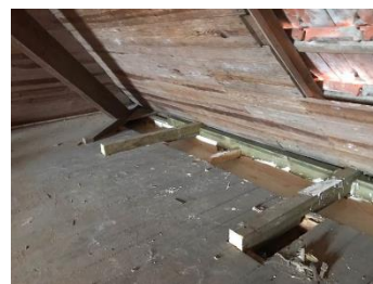
Figure 9. Splice of wooden beams (credits: Aníbal Costa)
