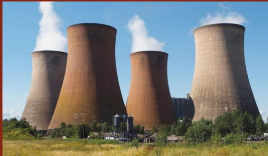
Torre de arrefecimento (The Spectator, 2021)
