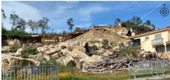
Fig. 2 Front view of the failed slope.
