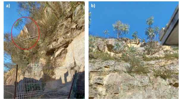
Fig. 8 Presence of potentially detachable blocks at risk of falling on slope sections 11 and 12.
