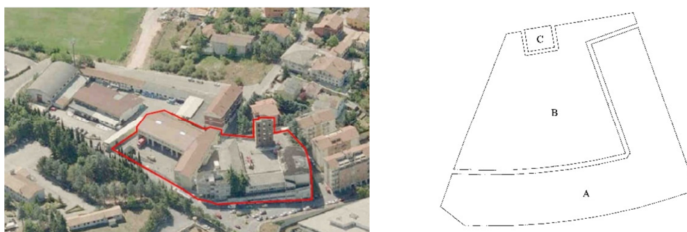
Fig. 1 - Aerial view and plan diagram of the complex object of the intervention (A-Building; B-Square; C-Tower) from (Provveditorato interregionale,2012)
