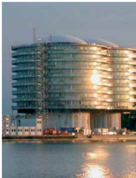
Fig. 6 - Example of deconstruction of old silos in Copenhagen for reconstruction for residential use
