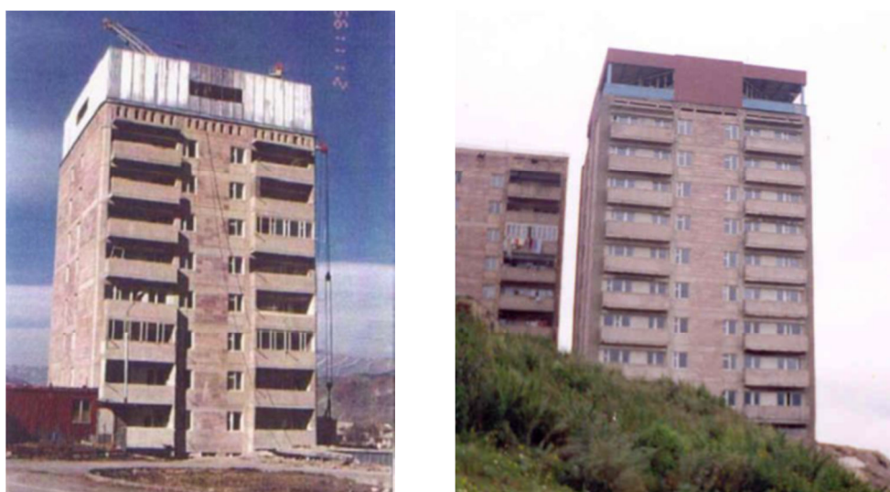
Fig. 5 - Seismic Upgraded Buildings using AIUF
