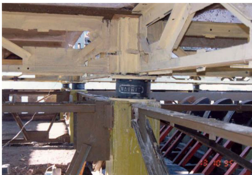
Fig. 6 - AIUF Implementation Technique on Roof Floor of 111 Series building
