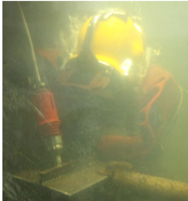
Fig. 2 - The process of underwater ultrasonic peening by using UltraPeen® system
