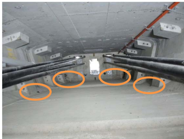
Fig. 4 Accelerometers inside bridge girder in Test 2.
