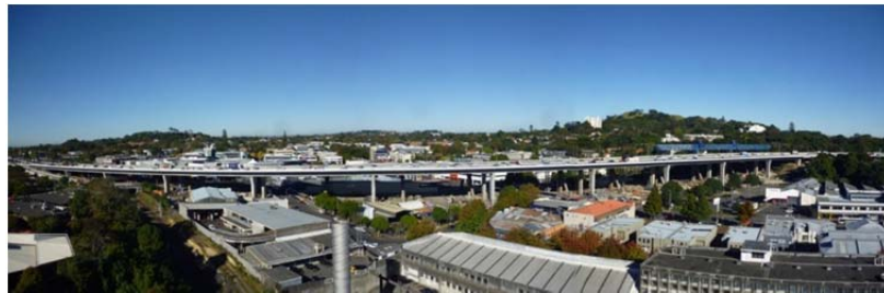
Fig. 2 Side view of Newmarket Viaduct.
