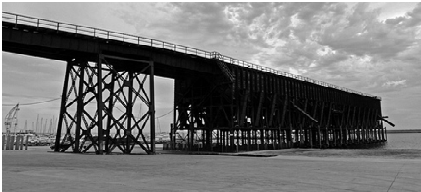
Fig. 1 - Lateral view of “El Cables Ingles” structure.
