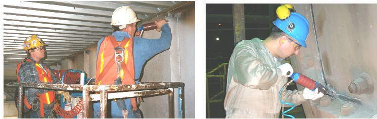
Fig. 1 - Application of UP for rehabilitation of welded elements in a welded bridge (left) and of a large grinding mill (right).
