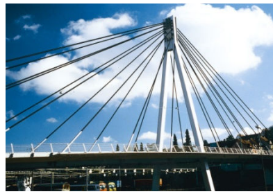
Fig.2 - CFRP cable stayed Stork Bridge in Winterthur crossing 18 tracks of the Swiss Railways
