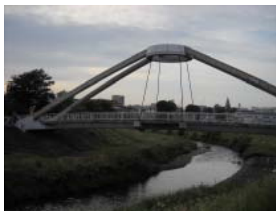
Fig. 1 Prime member in recent structure
