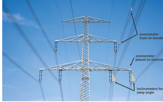
Fig. 3 Overview of measurement equipment around suspension tower
