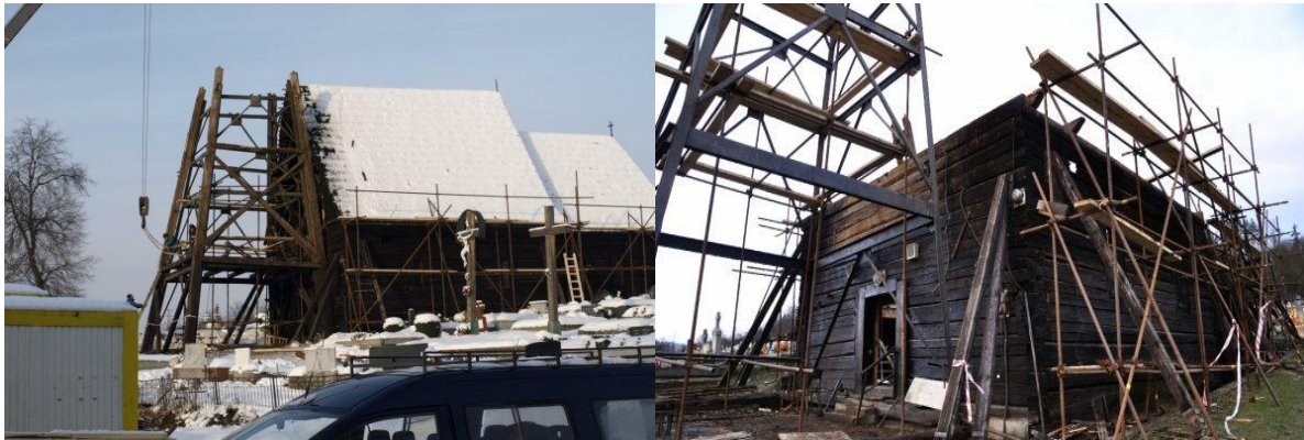
Fig. 3 Dismantling the wooden church
