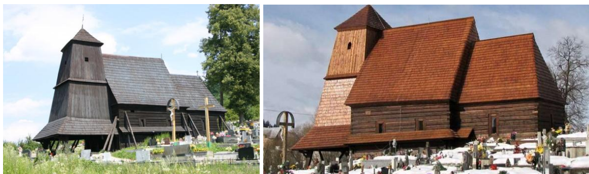
Fig. 9 Wooden church in Trnove On the left prior to reconstruction, on the right after reconstruction
