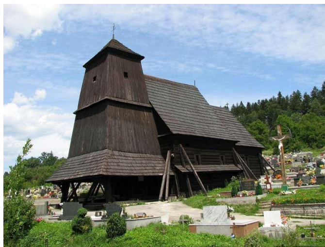
Fig. 1 Church of St. George in Zilina prior to reconstruction works
