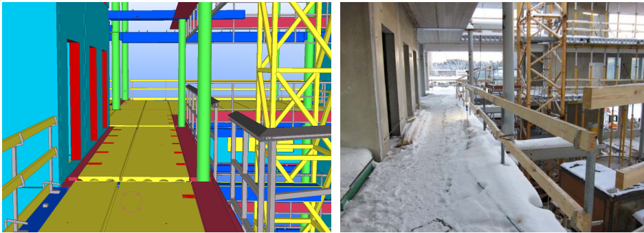
Figure 48. Comparing model and live situation: The final handrails of the building were intended to be used as falling prevention in construction phase.
