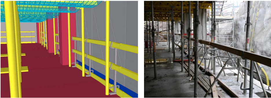
Figure 44. Comparing model and live situation: Safety railings in the slab edge in the second basement floor.
