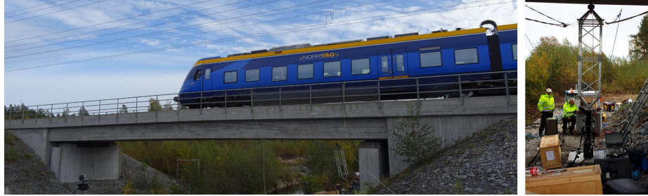
Fig. 1: Side view of the single-span railway bridge and the hydraulic actuator.
