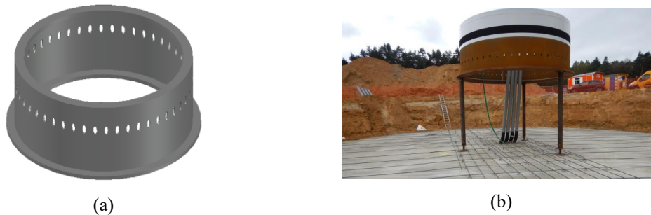
Figure 2. Connection between steel tower and concrete foundation using the TFS solution: (a) schematic drawing (b) onsite installation.
