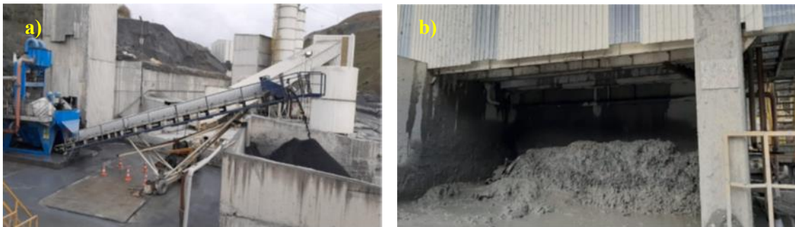
Figure 1. (a) Washing system and (b) Aggregate washing sludge pile.
